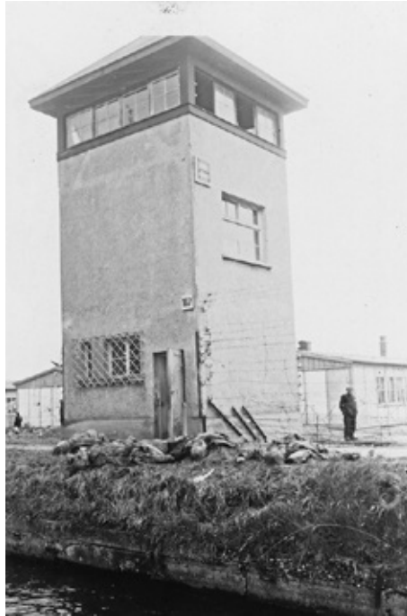
SS guards killed by American liberators lie beside a guard tower at Dachau concentration camp. [National Archives]
